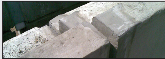
REPAIRING AND BEDDING CONCRETE
